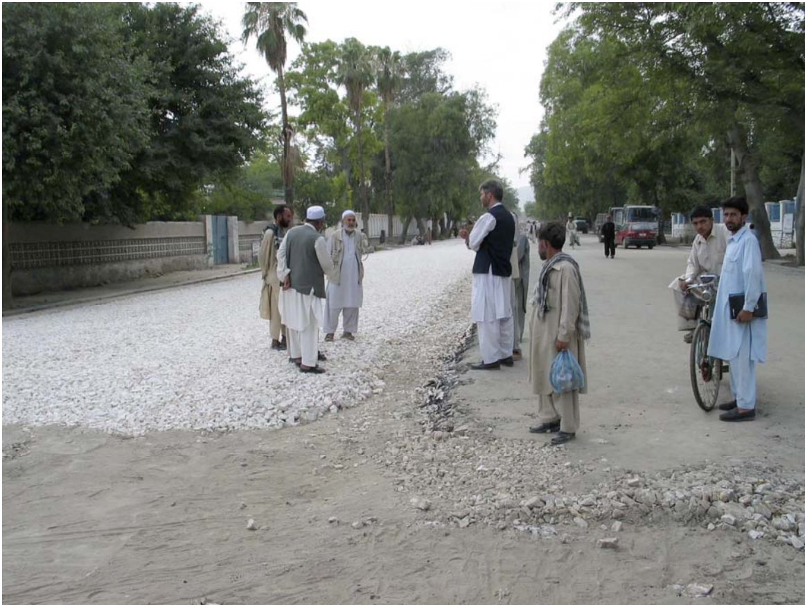
New road paving funded by the City.
