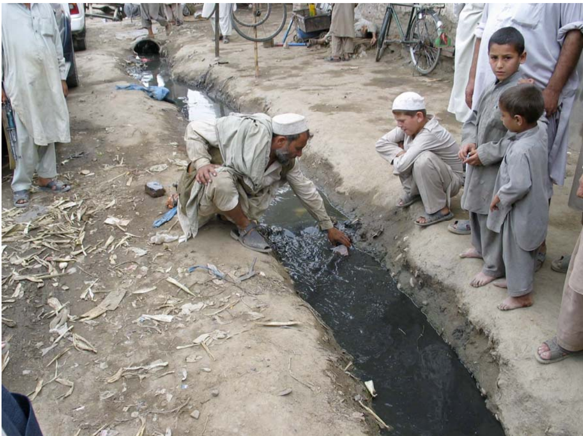
Drainage channel that remains after irrigated land has been converted to urbanized uses. The problems described previously, of a high water table, sewage overflows and the mixing of irrigation water and sewage exist because former irrigated agricultural areas are now part of the City.
